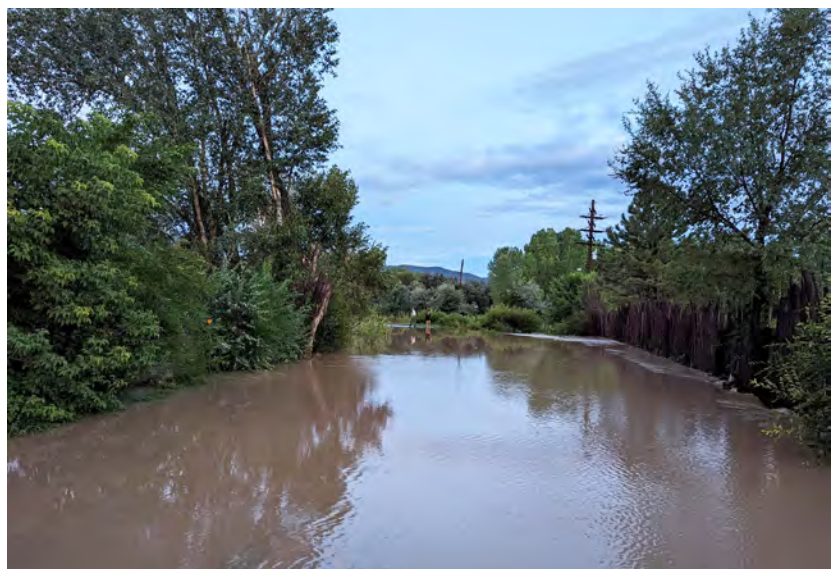
Road closure on NM 240 due to flooding in 2022. Source: NMDOT.
