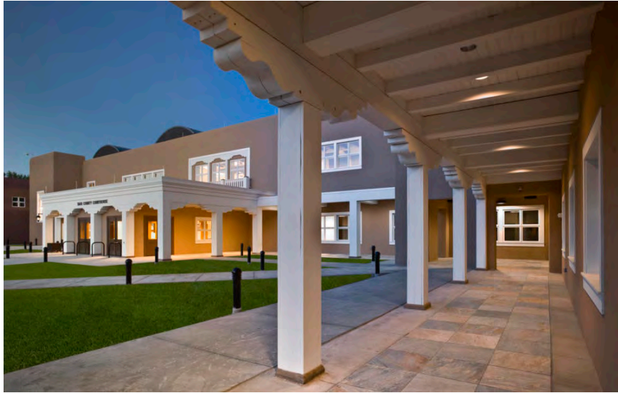
Taos County Judicial Complex. Source: HB Construction.
